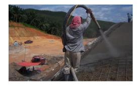
GZ-3A dry mix shotcrete machine/gunning machine is small-sized shotcrete machine for the dry spraying process.GZ-3A shotcrete machine can be used as well for small jobs, such as joint filling, swimming pool, refractory application and extensive slope consolidation work, etc.
