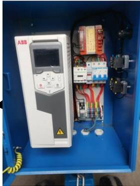
ABB variable-frequency drive/ABB 变频调速
