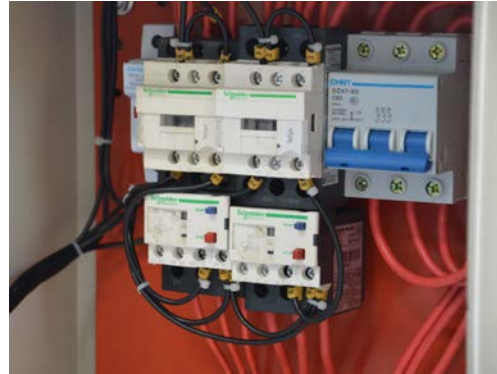
electrical control box for mixer and Agitator
