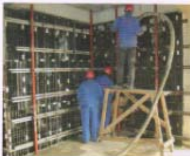
泡沫砼墙体浇筑 Cast-in-place foamed concrete wall
