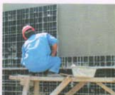
拆模板 Removing of mold
