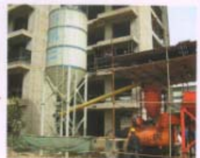
泡沫砼拌制 Foamed concrete mixing
